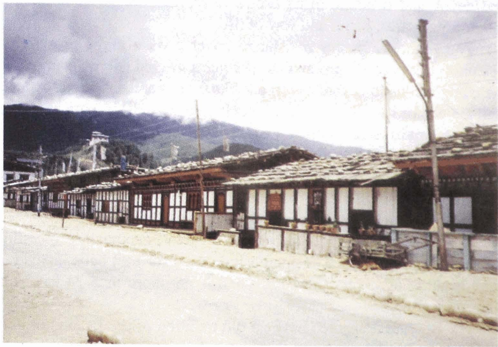
Plate 17 : Residential houses-cum-shops in Bumthang town
